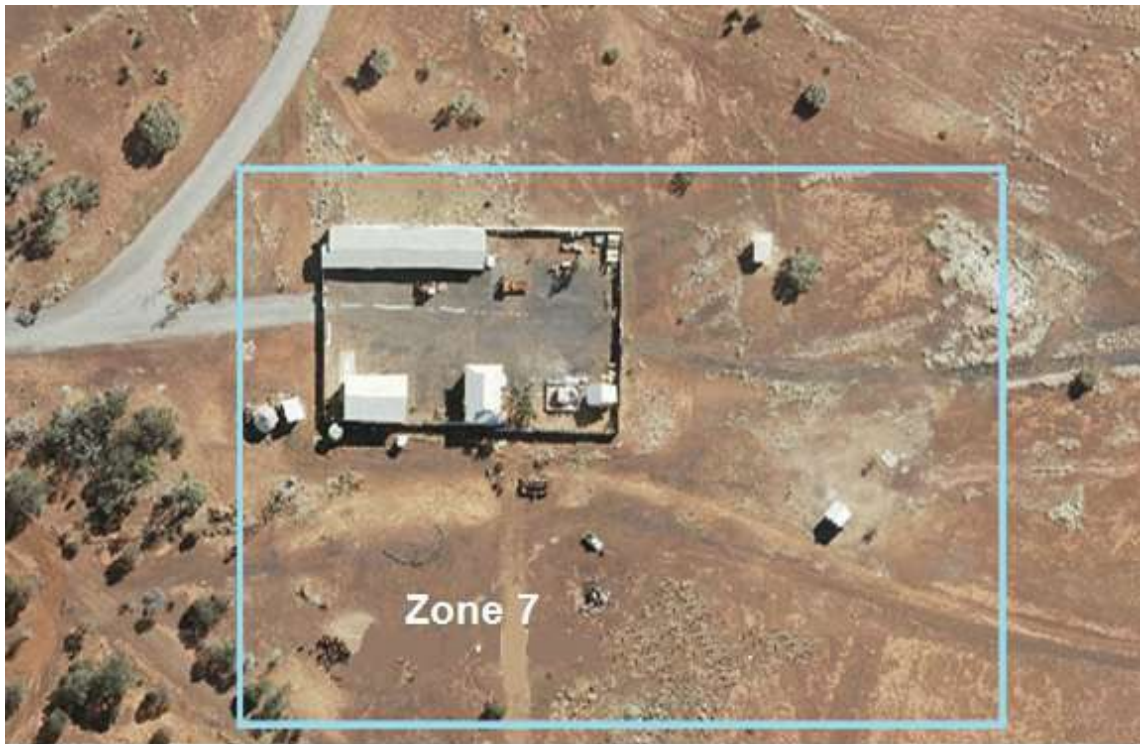
Figure Q – Zone 7 - Works Infrastructure
