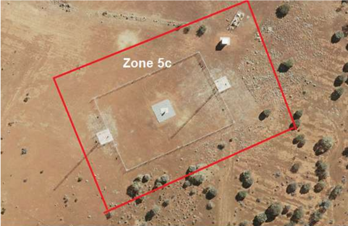
Figure N – Zone 5c - Communications - Non Directional Beacon
