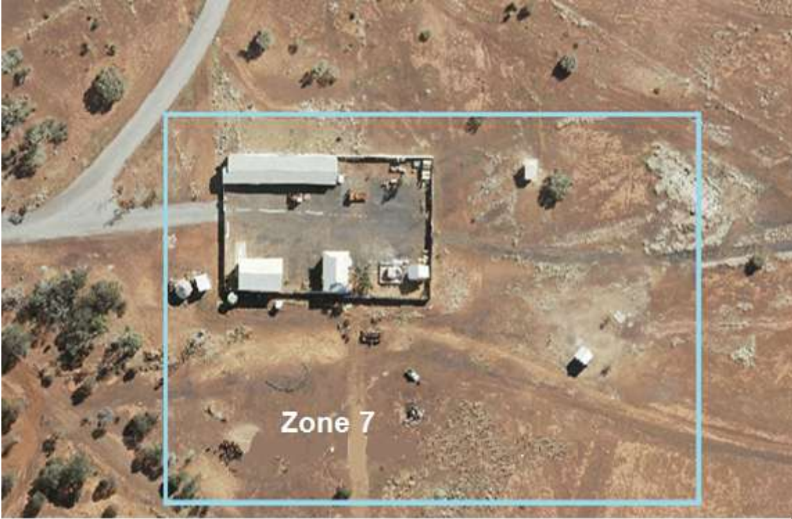
Figure Q – Zone 7 - Works Infrastructure
